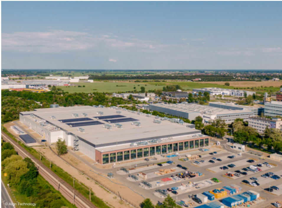
Align Technology's first Europe, Middle East & Africa (EMEA) regional manufacturing facility in Wroclaw, Poland (Photo: Business Wire)
